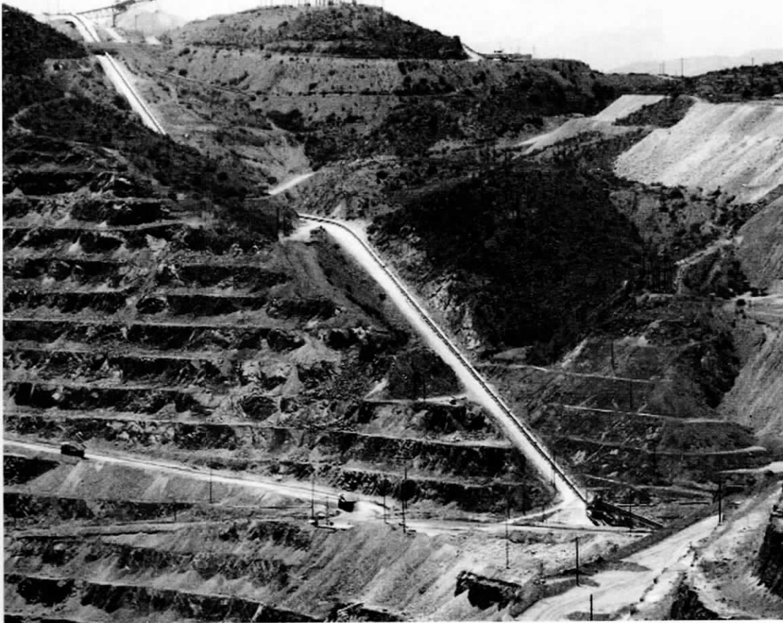
Figure 5. Ramp conveyor at a copper mine, Arizona. The difference in inclination between a truck ramp and an IPCC conveying ramp is clearly visible
